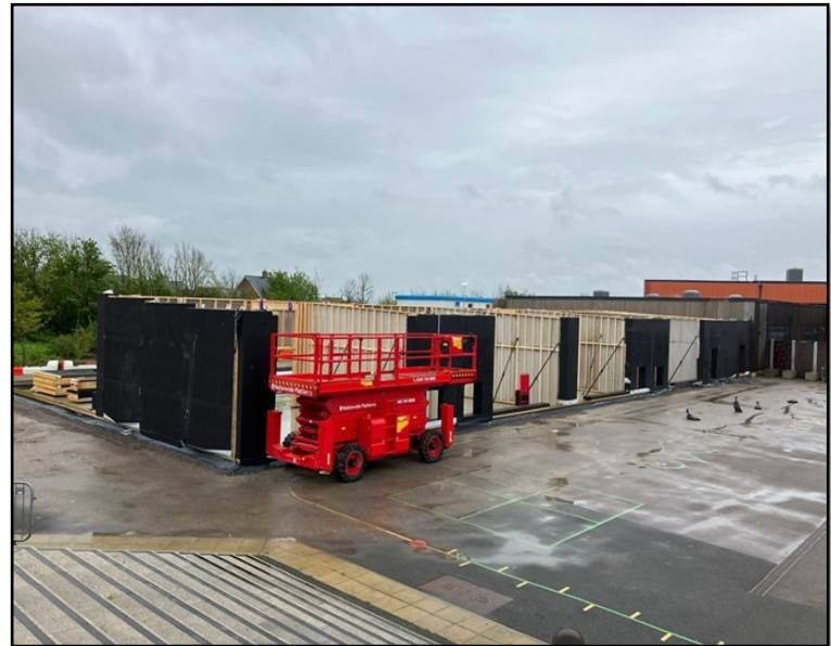
Fig 1.1 SIP's panels being installed to Green Ridge
