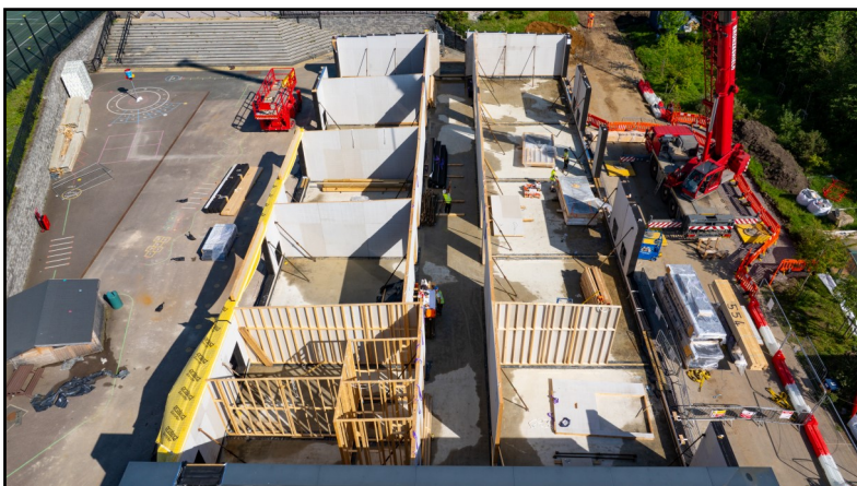
Fig 1.2. External New Build Extension
